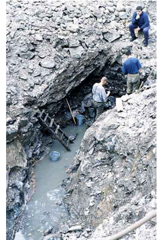
The open cast permanent works
